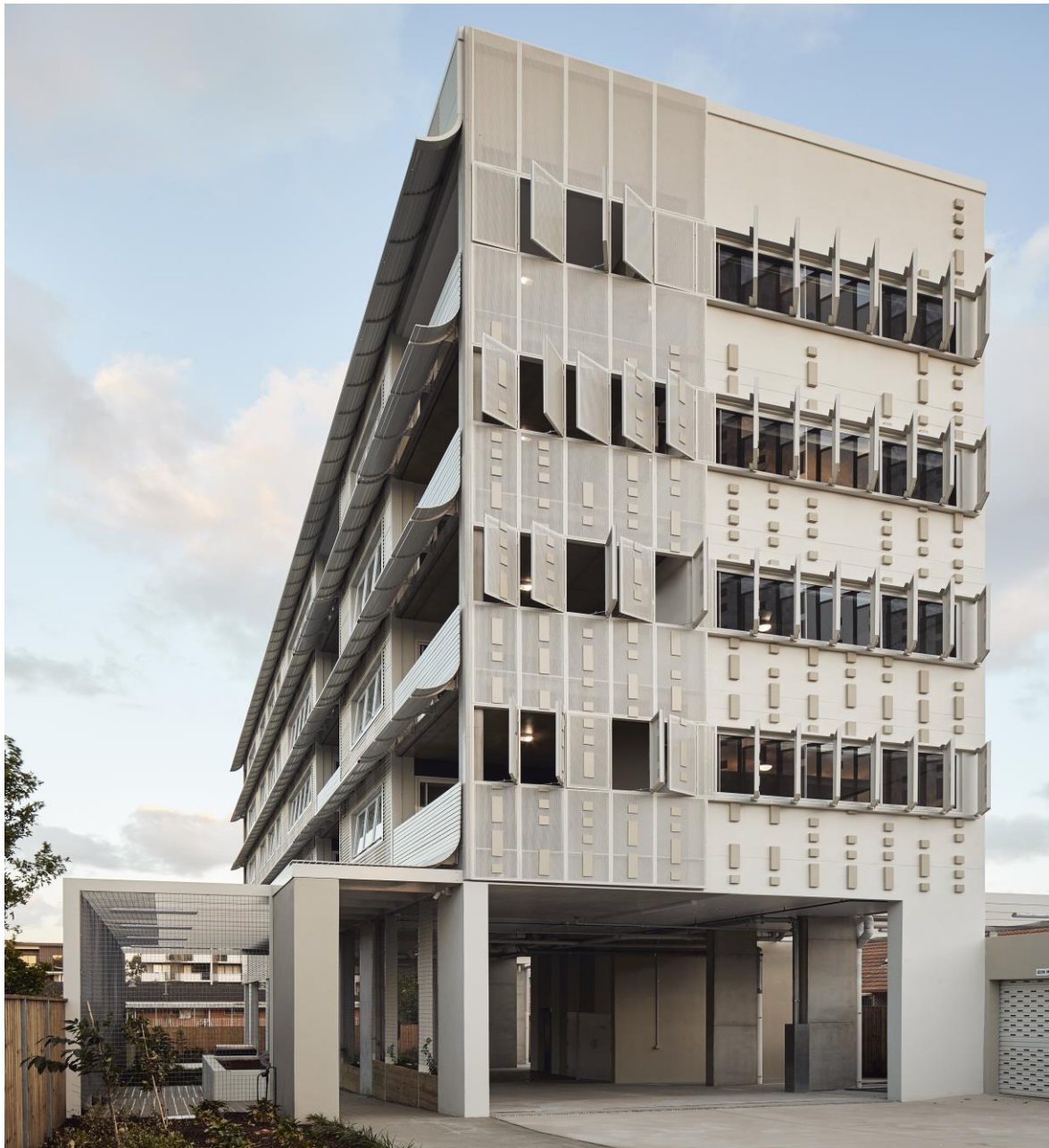
The Trust's apartments at 32 Primrose Street, Sherwood, Qld
